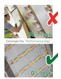
Make insulation great again – We all know that insulation is under performing and at times failing. By continuing to ignore the issue, the problem won't go away. Gapotape is here to help! When Gapotape is installed, it expands and pushes off the board, filling all the microspaces between the board and the rafter/stud/block/metal. Gapotape aims to improve the thermal performance of the insulation by x5, allowing for 0% loss.
