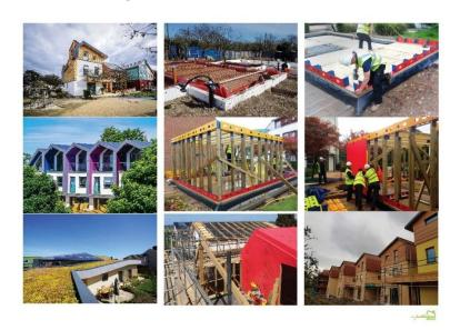
A low cost, zero carbon building designed to be modern and contemporary; built from locally sourced, traditional materials, combined to create a high performance, low environmental impact construction system. The system combines an energy efficient timber frame structure with an integrated solar PV roof.
